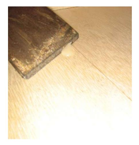
Remove all glue from the assembly frames. Use a **blunt** tool. **Please do not damage the frames!**
